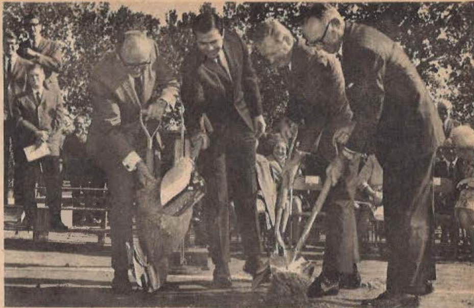
SHOVELS OF SAND fly as construction begins on the Walsh Medical Center at Southwestern Theological Seminary. Participating, left to right, are seminary President Robert E. Naylor, Student President Charles Lloyd, Contractor Herman Smith and F. Howard Walsh, seminary trustee, for whose family the new structure will be named. (Photo by Dave Clanton)
