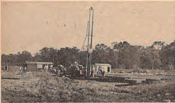
Laying Foundation Piling for Four Buildings, Fifty Family Units
