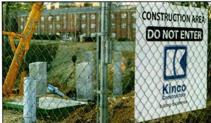
groundwork for the bridge is prepared by digging into the hill of the ravine. The support beams of the bridge were placed in early fall.
