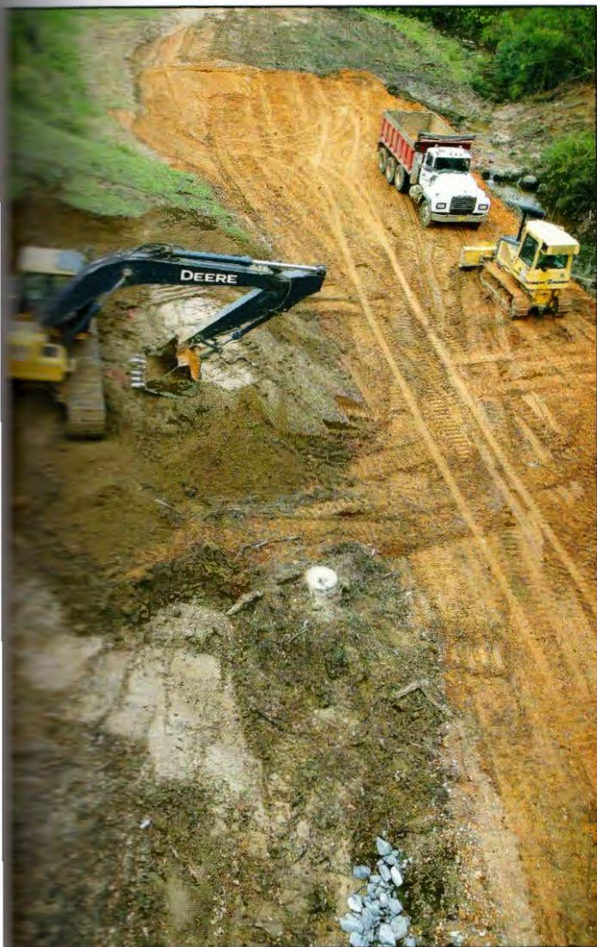
Groundwork for the bridge is prepared by digging into the hill of the ravine. The support beams of the bridge were placed in early fall.
