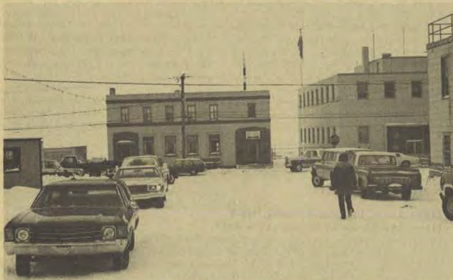
Behind these buildings in downtown Nome is the Bering Sea.
