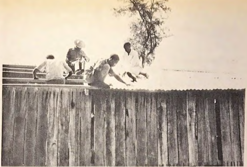
Church members add a tin roof to the walls of the church they have built from lumber cut nearby and hewn with a crosscut saw. It replaces a mud building with a grass roof.
