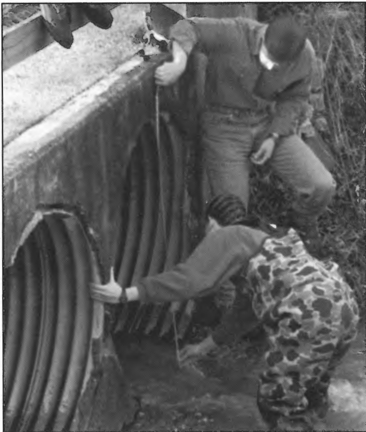
MEASURE UP Senior Marcy Franks and Dr. Knight measure a culvert. The area of the culvert determined the stream of the flow of the water. •photo by John Barber
