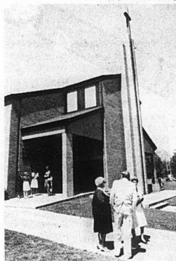
First Church, Nashville's present sanctuary, constructed in 1969, is the third worship facility for the congregation in its 150-year history.
