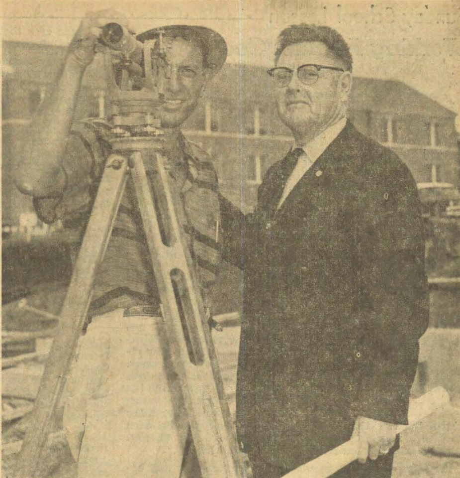
SURVEYING THE FUTURE: Looking over the site of the Oklahoma Baptist University Memorial chapel are Pete Veitenheimer, Jr., carpentry foreman, and Dr. John W. Raley, University president. Cash and pledges for the million dollar building have reached $542,785.88, enough to start the second stage of construction. ■
