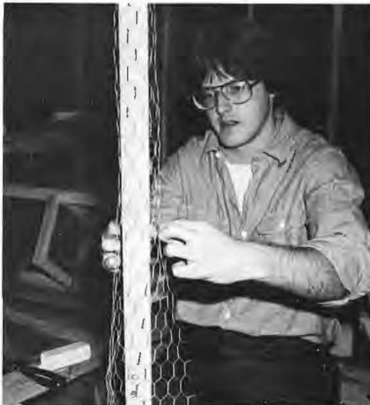
ZETA BEAU TERRY DANIELL begins the tedious job of covering the
