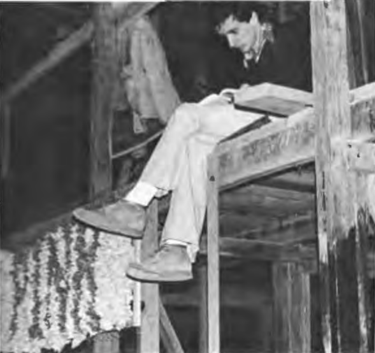
squeezes in a little studying at the float building site. A Hardman Lumber Company warehouse was used instead of the usual fairgrounds.
