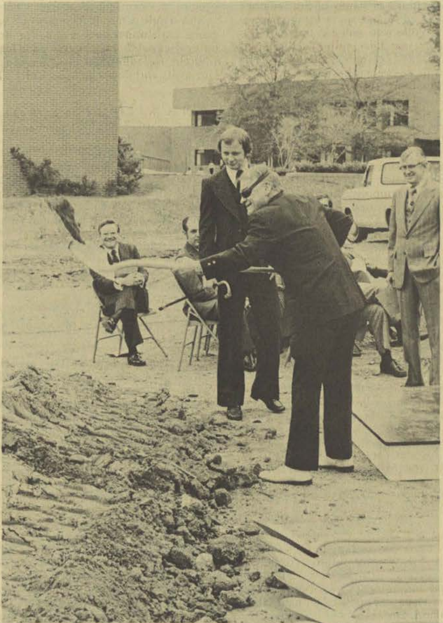
GROUND BREAKING — Bob Riley, chairman of the Political Science Department at Ouachita, tosses a shovelful of dirt during groundbreaking ceremonies on the site of McClellan Hall. Mark Lowman, a political science student, stands directly behind him. Also looking on are Ben M. Elrod (seated), vice president for development; Roy Lewis, associate executive secretary-treasurer of the Arkansas Baptist State Convention; and Daniel R. Grant (standing at right), president of OBU.
