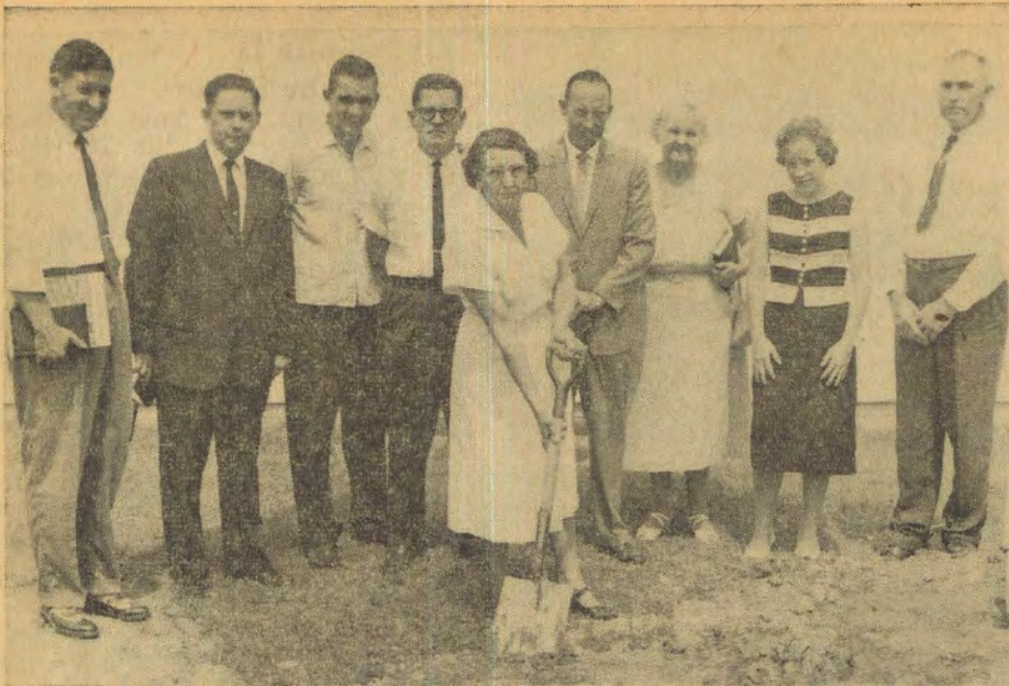
SPRADLING CHURCH held groundbreaking services Sunday, Aug. 30, for their new educational building which will provide for a total of 255 people. The approximate cost will be $32,000. Turning the first shovel of dirt is Mrs. Daisy St. Mary, one of the oldest charter members of the church. In the background, left to right are: Fay Hobbs, chairman of deacons; Rev. Paul Graham, pastor; Gorman O'Neal, Training Union director; Lee White, treasurer; S. R. Kennedy, Sunday School superintendent; Mrs. A. G. Gilson, WMS president; Miss Janette Orr, youth fellowship president; and Edgar Rozell, chairman of the Planning and Survey Committee.
