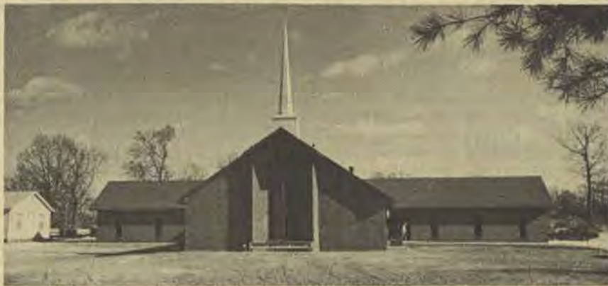
Huntsville Church's new auditorium and education building are valued at $145,000.
