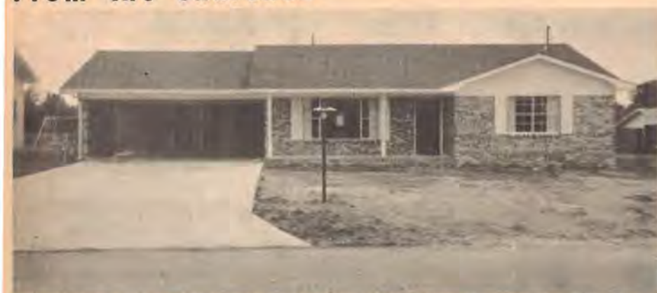
DANVILLE First Church recently completed this Gold Medallion parsonage for its pastor, Carl J. Pearson. The home contains 1,718 square feet, central heat and air conditioning. It features three bedrooms, two baths, a family room, kitchen, dining area, living room, study and double carport.
