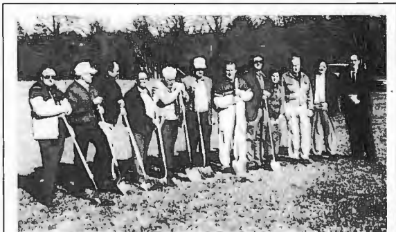
First Church of Jasper broke ground Nov. 12 for a 12,500-square-foot worship center at its new location site on Scenic Byway 7. The concrete slab has already been poured for the 250-seat facility that will be constructed in the spring by a volunteer group from Texas. The old church property has been sold to adjoining Jasper Public School. Those participating in the ceremony were (left to right) Ed Wilhoit, Harry Moore, Richard Waters, Fred Bell, Bob Jones, C.B. Hudson, county judge Eugene Villines, mayor Shannon Willis, Virginia Lavery, Bob Magennis, North Arkansas Association director of missions Royce Sweatman and pastor Manuel Macks.
