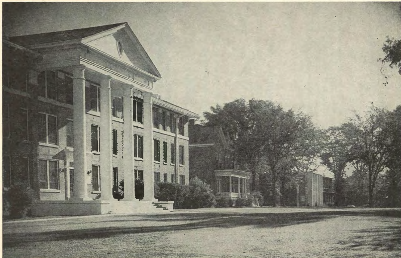
South View of Campus Showing Cone-Bottoms Hall, The Mansion, and J. R. Grant Memorial (Administration Building)
