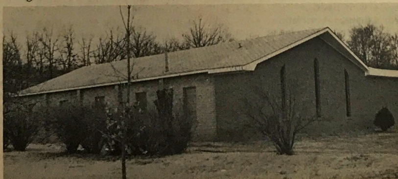
Sang Avenue Mission's building was bought from another denomination.
