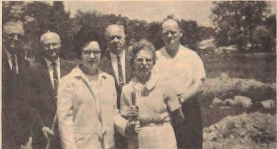
NORTHSIDE Chapel, Eudora, broke ground May 5 for a new 250-seat auditorium, which they hope to have completed by early fall. The hadite-brick structure will be the first unit in a three-unit building. It will consist of seven new Sunday School rooms, a baptistry, pastor's study and secretary's office. The church membership numbers 187. Shown here, left to right, front row: Mrs. Peggy Jones, music; Mrs. Eugie Harrell Sr., WMU; back row, left to right: the pastor, Leslie J. Ready; J. P. Cheatham Sr., building committee chairman, Gaines Morgan, Edd Britton. N. L. McDuffie, another building committee member, was not available when the picture was taken.
