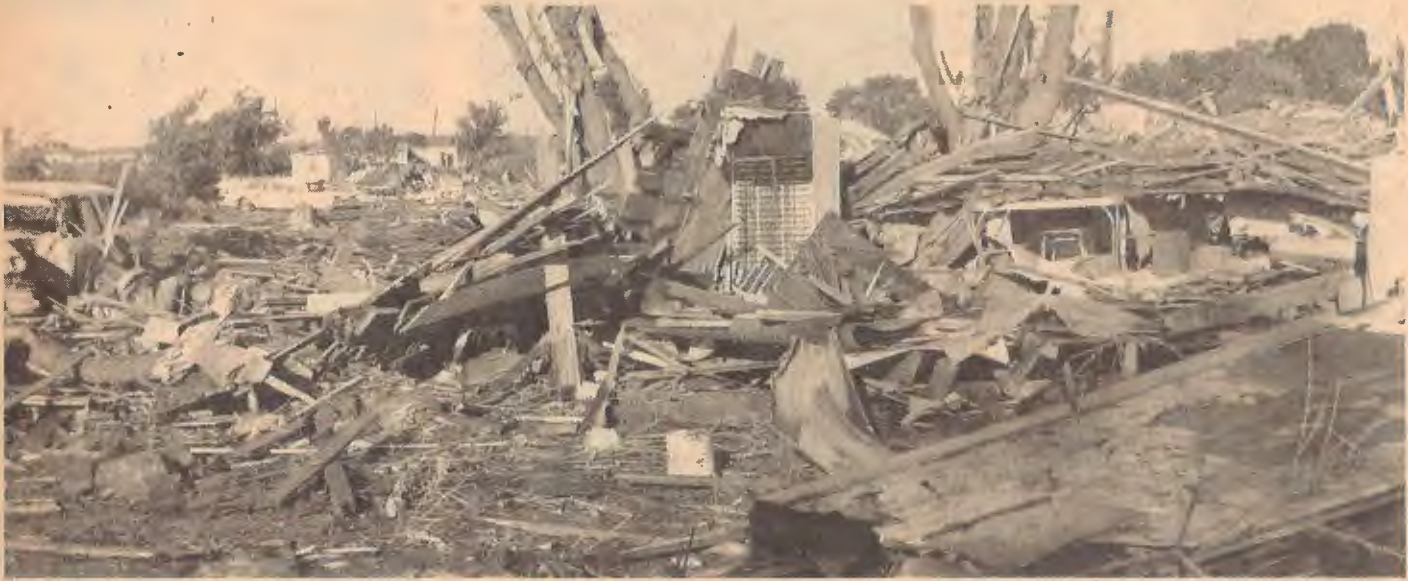
WE were unable to identify whose house this was, but it is a typical picture of the disaster.
