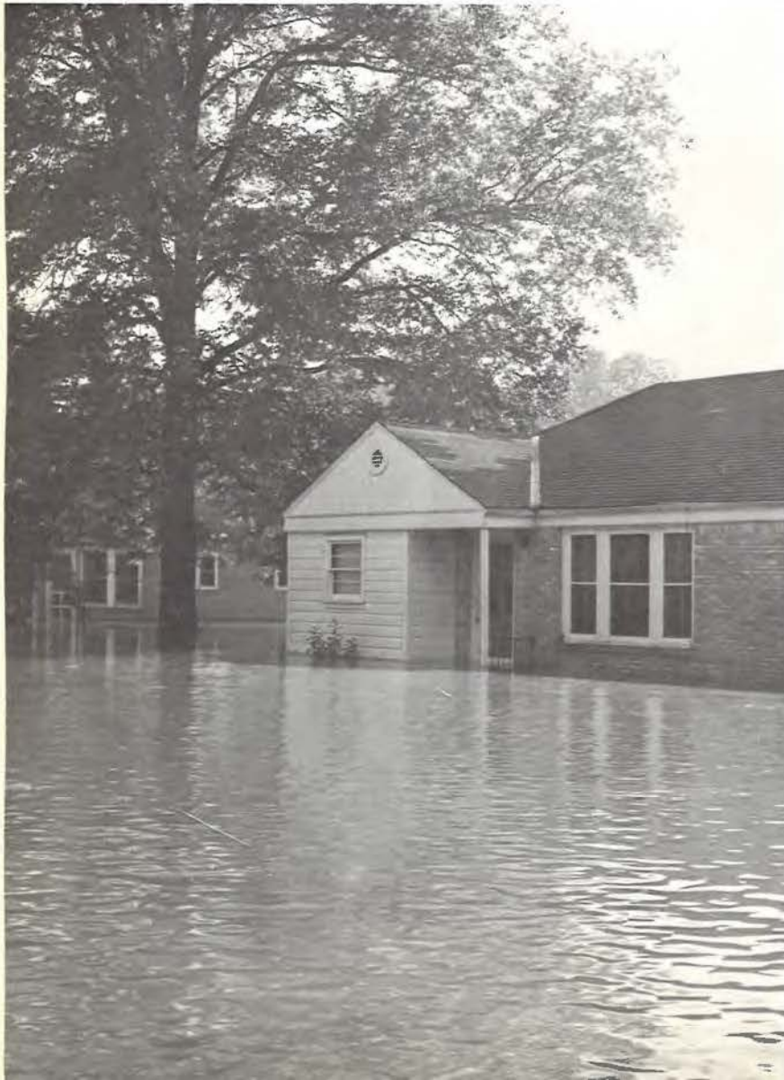
Residents of North Campus found their apartments filled with water during the May flood.
