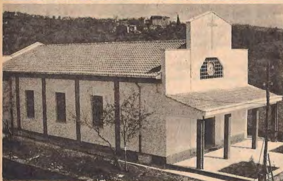
NEARLY 10 years after construction first began, Baptists of Sant'Angelo in Villa, Italy, recently dedicated this church building. A village of about 400 people, Sant'Angelo is set among vineyards and olive groves approximately 50 miles from Rome. About half the villagers are Baptists. (Photo by Frederick H. Anderton)
