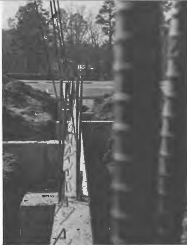
Concrete and steel began their growth into the new men's dorm.
