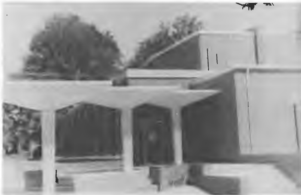
Newly completed Verser Speech and Drama Center offers modern facilities for play production.
