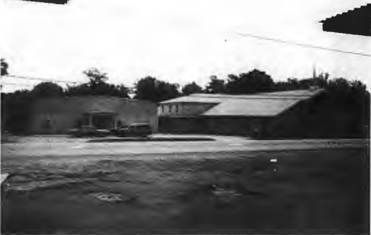
White Hall First Church dedicated new facilities May 17. The new 10,220-square-foot facility, with an insurance value of approximately $263,000, was constructed at a cost of $205,676 because numerous volunteers assisted in construction. The building, dedicated debt-free, was erected as funds became available with the church doing its own fund-raising program. The new facilities house five offices, a conference room, four Sunday School rooms, two bathrooms, and a multi-purpose space. This space is designed for a fellowship ball that will seat 400 people, a basketball and game area, and a large kitchen. The dedication service included recognition of all who had assisted with construction. Pastor Bob Harper brought the dedicatory message. The evening service featured Gerald and Catherine Taylor, missionaries to Senegal, who served the White Hall church when the present sanctuary was erected.
