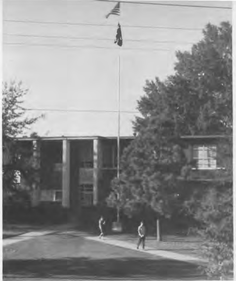
The offices of the administrative staff are found in the J.R. Grant Memorial Building.
