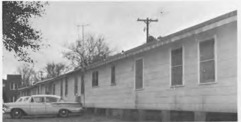
Lakeside. Temporary men's quarters.
