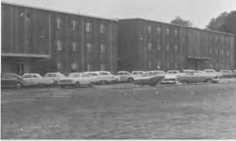
West-Northwest. Newest men's living facilities.
