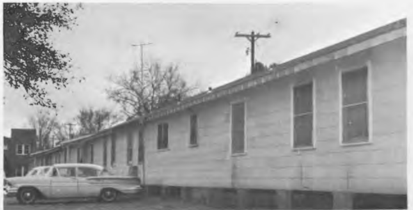
Lakeside. Temporary men's quarters.
