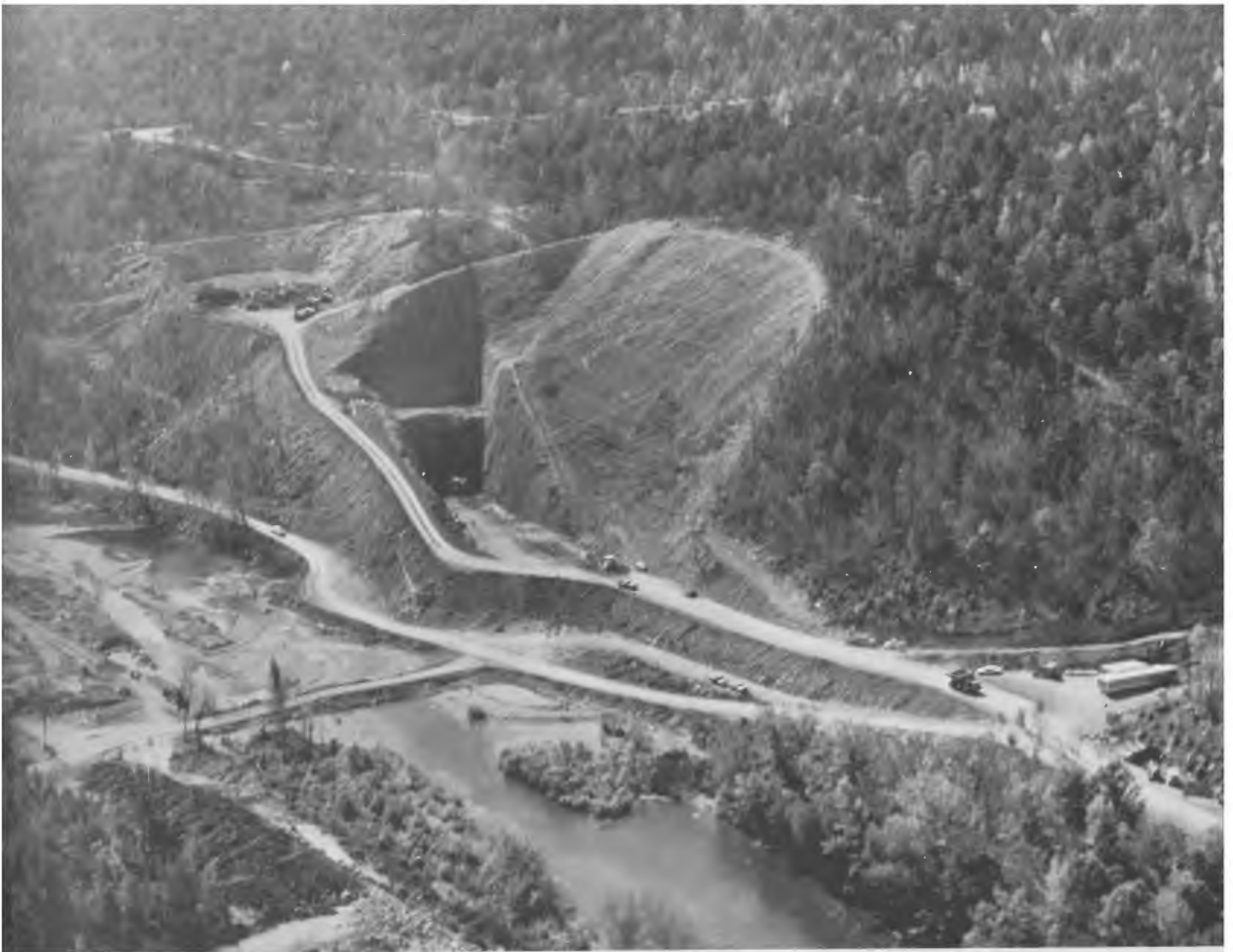
Extending 243 feet high, and costing $50 million, the DeGray Dam, under construction by the U.S. Corps of Engineers, is a multi-purpose dam and reservoir which will provide flood control, hydro-electric-power, industrial water, and recreation when completed.
