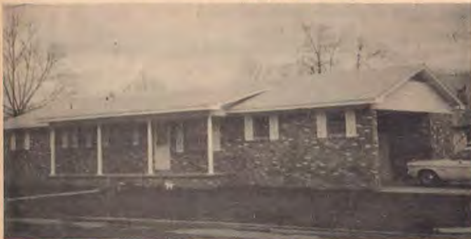
PARAGOULD'S Immanuel Church recently completed this parsonage for its pastor, Rev. Eugene Ray. The $20,000 structure contains four bedrooms, two baths, a family room and a double carport.
