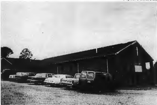
The Belview Church, Melbourne, dedicated its new 11,600 square foot facility April 26. The facility was erected at a cost of $200,000, but has a replacement value of approximately $400,000. The building was constructed with the help of the Arkansas Nalibenders and other volunteer labor. The auditorium will seat 320 people and the building contains 14 Sunday School rooms, a fellowship hall and kitchen, a nursery, a prayer room, a library/conference room, and three offices. The auditorium is fully carpeted and has a baptistry. The facility has central heat and air. All of the windows are tinted and the picture window behind the baptistry is constructed with a cross. Tim Porter is pastor.
