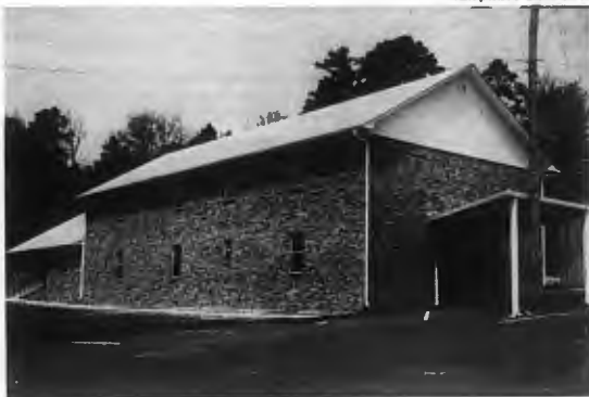
Martindale Church, Little Rock, held a dedication for their new educational facility April 12. The old building burned in July of 1989 and the insurance paid for the new building that was erected at a cost of $120,000. The building houses the pre-school and children's departments and contains 6,000 square feet. It has 10 Sunday School rooms, a choir room, four restrooms, a pastor's office, and a secretary's office. The two-story facility is carpeted throughout and has central heat and air conditioning. In addition to the new construction, a 20-car paved parking lot was dedicated. Siding also was placed on the fellowship hall and additional drains were installed. Pulaski Association Director of Missions Glenn Hickey was the dedicatory speaker. Scott Johnson is pastor. The dedicatory was followed by an open-house.
