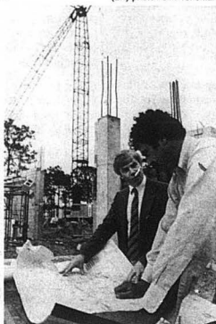
Checking over the plans.
