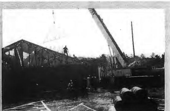
Arkansas Baptists' Church in a Day team, led by chairman Bob Fluharty of Little Rock and coordinator Ronnie O'Neal of the Arkansas Baptist State Convention's Brotherhood department, traveled to Perryville Sept. 5-6 to construct a new church facility for Second Church. The team, assisted by several Texas volunteers, built a 5,440-square-foot facility that will house an auditorium with a seating capacity of 200, classrooms, a fellowship hall, kitchen and nursery. Gifts for the building program have been provided by church members, friends, the ABCS missions department and a Texas foundation. Jim Haggard is interim pastor for the church which has been meeting for 15 months in a tailgrounds building.
