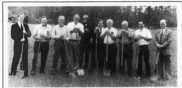
Westside Church of Warren recently broke ground to reconstruct worship and educational facilities destroyed by fire Jan. 18. Completion of the new facilities is scheduled for November. Lonnie Latham, director of missions for Bartholomew Association, and Jimmie Sheffield, associate executive director of the Arkansas Baptist State Convention, were speakers for the service. Breaking ground were (left to right) Latham, Mickey Tucker, L.V. Mills, Ted Herring, Rusty Rowell, pastor Wally Ferguson, J.W. Hardin, Bob Clayton, Eddie Stiles and Sheffield.
