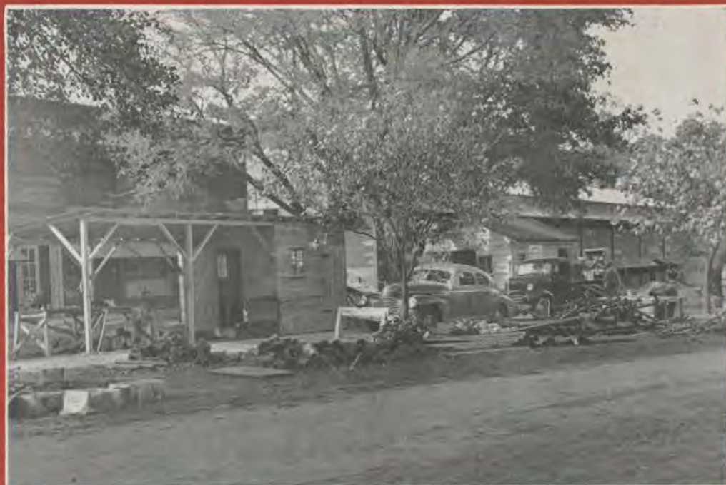
Construction On New Buildings
