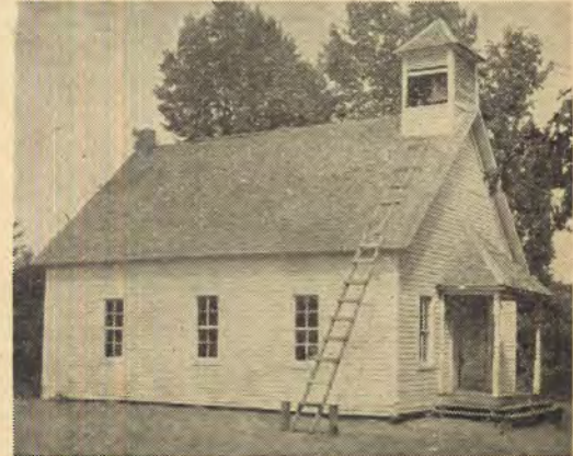
Old Church Building
