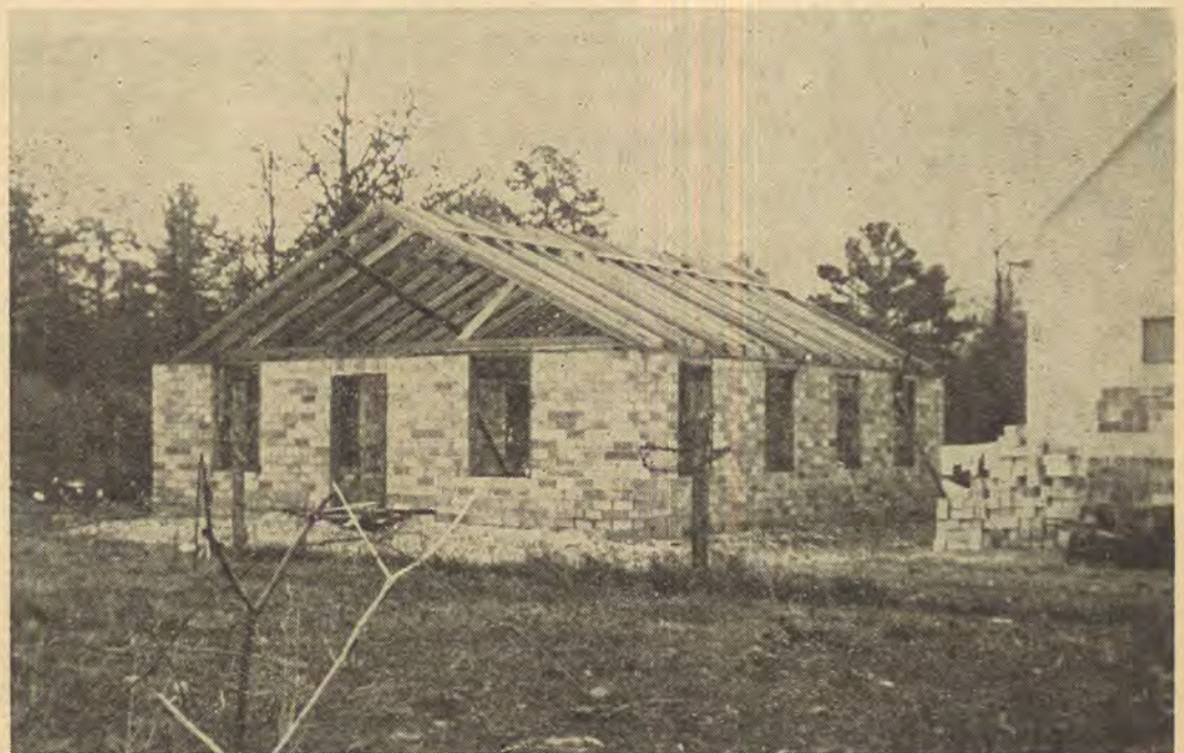
New Educational Building Under Construction
