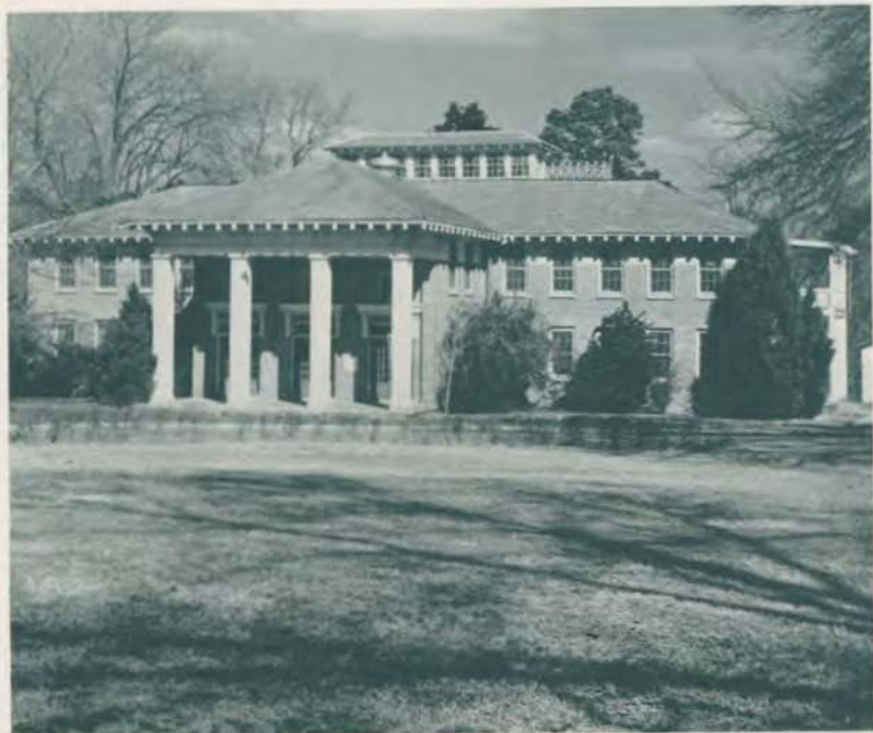
DINING HALL—FINE ARTS BUILDING
