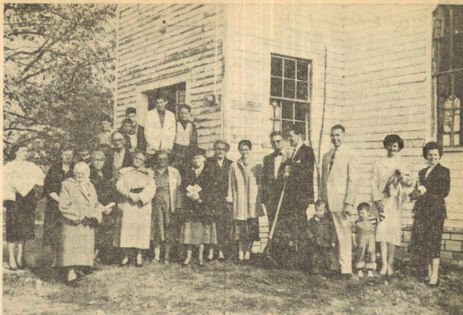
Ground breaking at Cushman Church.
