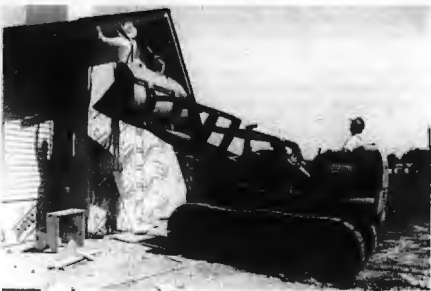
▲ Baptist volunteers from Texas and Alabama install trim on the new Ida Grove Baptist Chapel building. The church's ministry was aided by Oak Grove Church in Van Buren, which sent a Vacation Bible School team to the northwest Iowa town.
