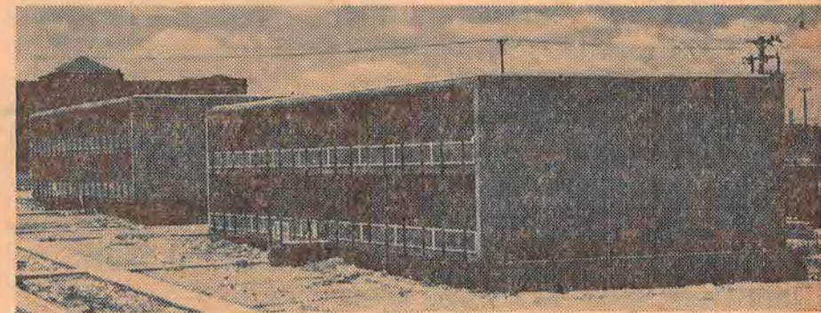
NEW STUDENT apartment unit at Southwestern Seminary
