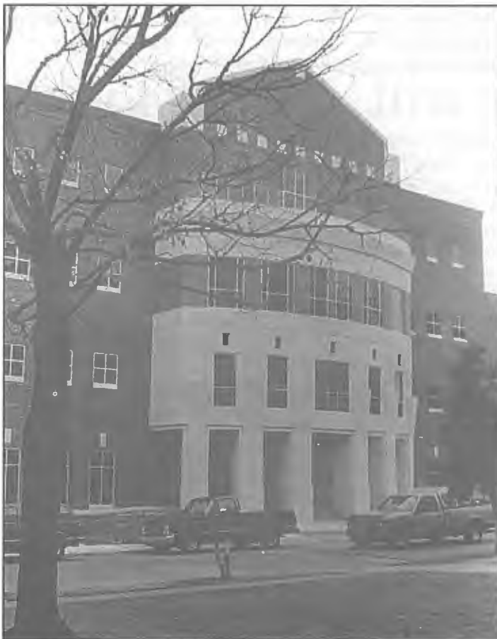
JONES SCIENCE CENTER • The Harvey Jones Science Center is complete and offices, classrooms and labs are in the process of being moved to the new facility.
