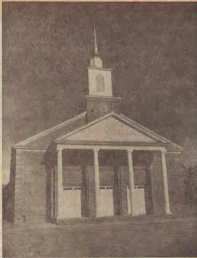
ELLIOTT Baptist Church held dedication services for this new auditorium and two new educational additions, on Sunday, Sept. 25. Dr. S. A. Whitlow, executive secretary of the State Convention, brought the dedicatory message. These buildings have been under construction for the past year and have been completed at a cost of approximately $70,000. The new auditorium is both centrally heated and cooled and will seat approximately 425.
