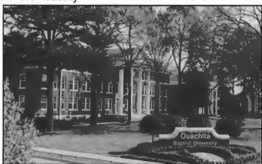
◆ The landmark Cone-Bottoms Hall, once a residence hall for women, returns to use as the university's administration building.
