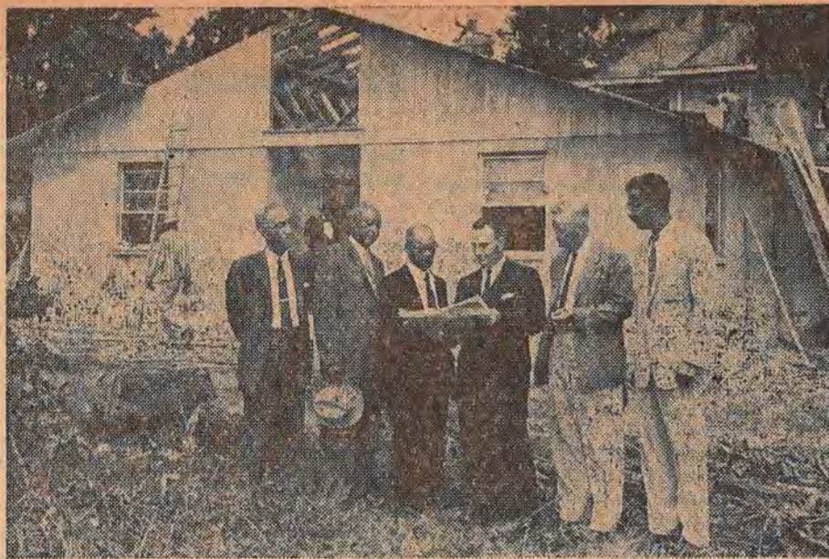
MEMBERS FROM the board of trustees of Arkansas Baptist College, Little Rock, confer in front of the new dormitory for men now under construction on the college campus. Left to right: Attorney J. R. Booker, Little Rock; F. S. Thomas, Batesville; Dr. Roland Smith, pastor of 1st Church, Little Rock; Dr. Dale Cowling, 2nd Church, Little Rock; Paul Mears, Dardanelle; and Oscar Rogers, president of the college.
