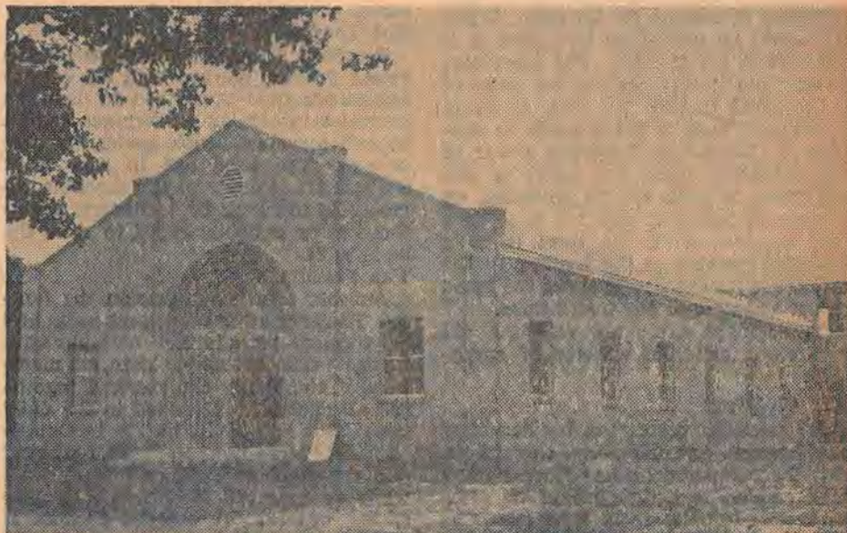
THE NEW building of South Texarkana Church was dedicated Sept. 14.
