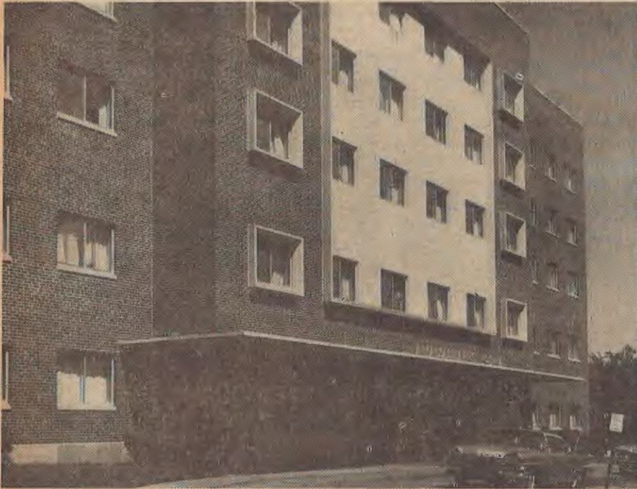
THIS is Arkansas Baptist Hospital today, where hospital care at its finest is offered to patients from throughout Arkansas.
