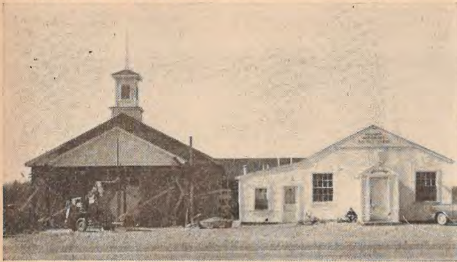
SHANNON CHURCH is completing its new sanctuary to minister to the needs of the people in the Pocahontas area.
