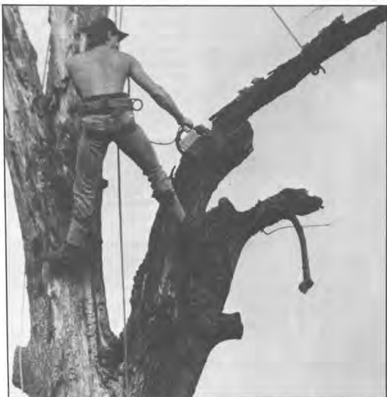
■ A tree service employee works from the top down in removing the century-old oak tree that stood in front of Evans Student Center. The tree, which was dying of disease, has been replaced by a fresh young oak.
