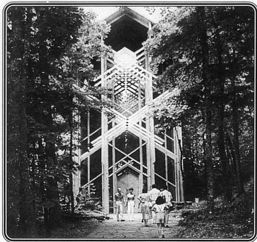
Thorncrown Chapel is noted for its award-winning architecture.
