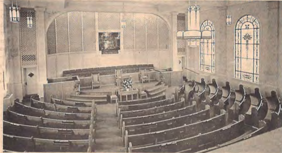
SANCTUARY of First Church, Paragould, which was renovated at a total cost of $36,890.
