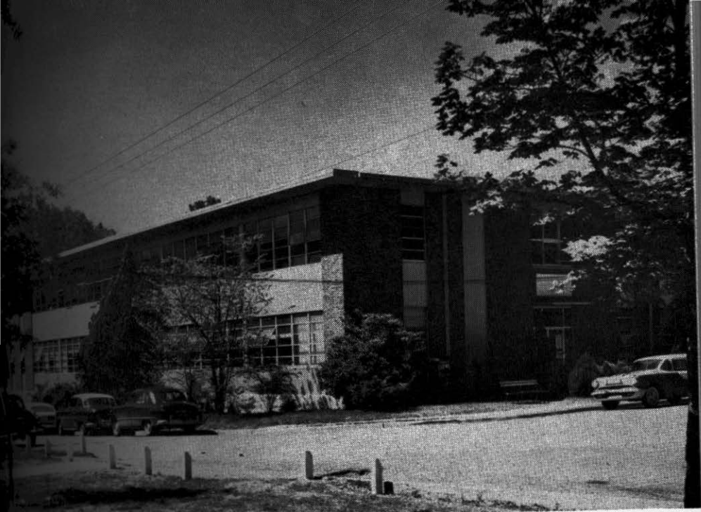
Hamilton Moses Science Building
