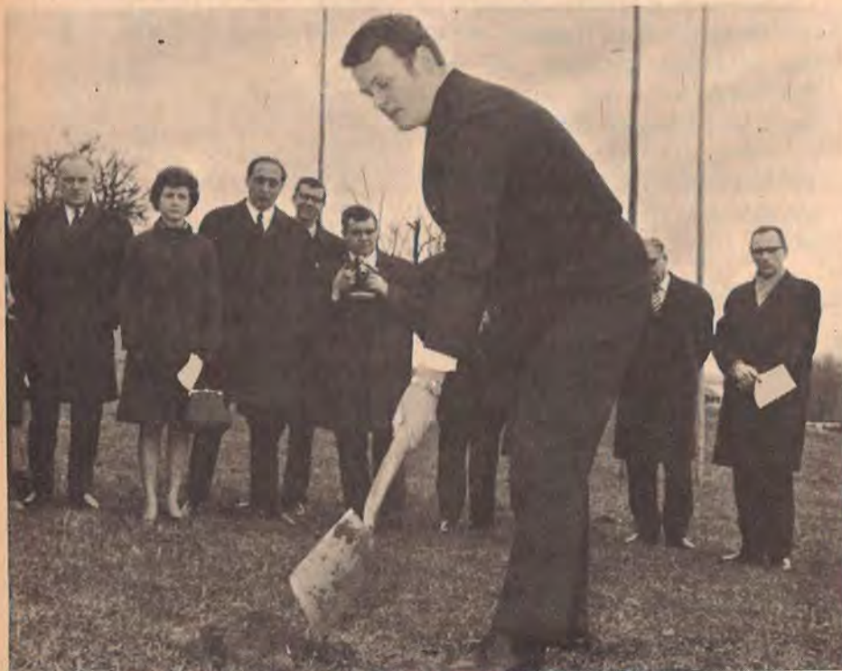
HARRY MAANSUS, Vasa, Finland, student body president at the Baptist seminary in Ruschlikon, Switzerland, breaks ground for the seminary's new apartment building. When completed early next year, the building will accommodate 10 to 12 married students and their families, meeting what seminary president John D. W. Watts considers an urgent housing need. It is the first seminary building that will not be located on the main campus; it is going up on Baptist-owned land ½ kilometer from the campus. (European Baptist Press Service Photo) Photo)
