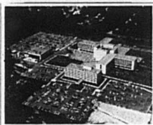
Baptist Memorial Hospital East 6019 Walnut Grove Road, Memphis
