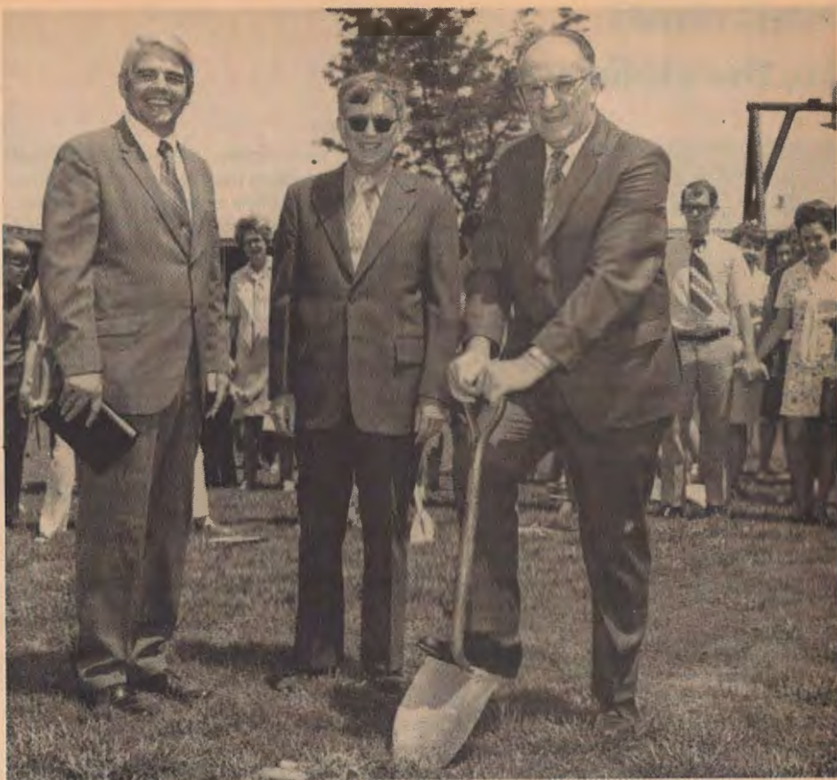
BEGIN BUILDING —Members of Harvard Avenue Church, Siloam Springs, broke ground last month for a new sanctuary. Pastor Bill Gray (left), Fred Olney, chairman of the Trustees, and Henry Hall, chairman of the deacons, took part in ceremonies. The building will contain 5800 square feet and seating for 330, plus a balcony. Plans call for exposed beams and decking with brick interior walls. Work is expected to be completed by the end of the year.
