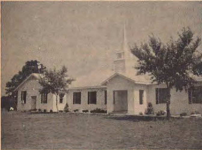
NORTHEAST CHAPEL, TEXARKANA — Assisting with building repair, pastor's salary and addition to property.
