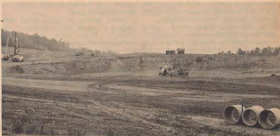
BELOW — The same approximate area is shown, 25 days after construction began.
